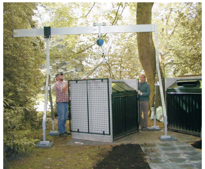
Positioning a garbage container
