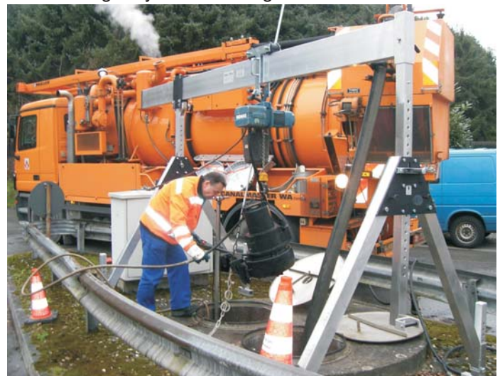
Maintenance work on a dirty water pump
