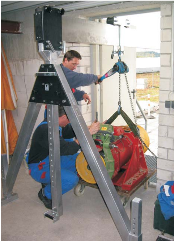
Withdrawal of a drive motor for a peoples' elevator
